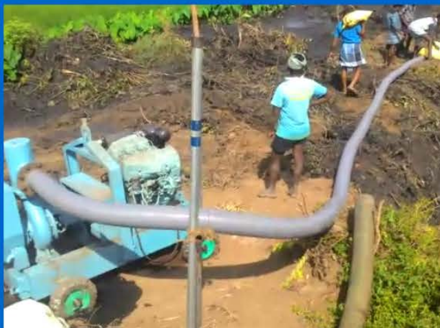
FLOOD AND DRAINAGE CLEANING
